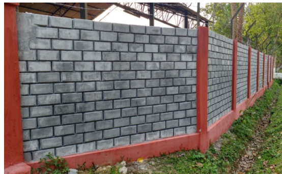
Photo: Modular Brick used construction of Boundary Wall at CSIR-NEIST, Jorhat
